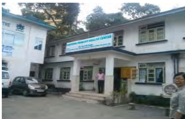
Figure 4: Front View of PHC Pakyong, East District
